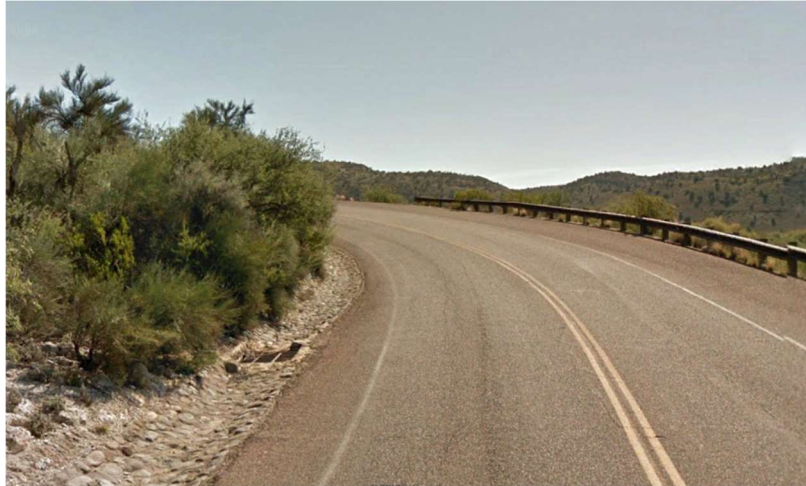
Figure 2: Stopping Sight Distance Example
